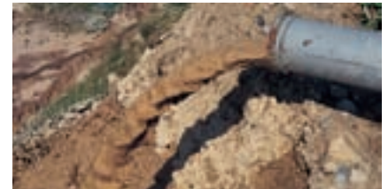
Removing slurry from a tunnel
