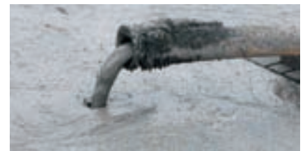
Pumping lime slurry
