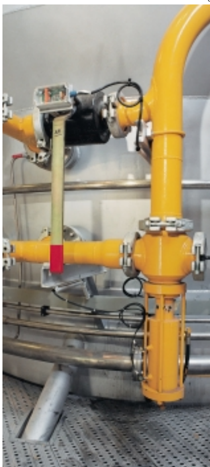
Sewage sludge being fed into a fluidized bed incinerator
