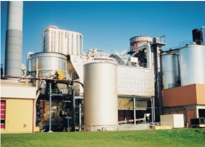
Sewage sludge reception station consisting of reception and storage silos: incineration of foreign sludges at the main sewage works in Stuttgart Mühlhausen
