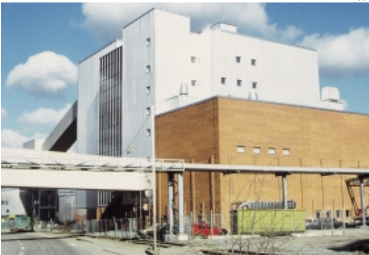
Clean air above and around the Värtan heating power station. The illustration shows the coal preparation plant with the coal transportation lines carried in the pipe bridge with inspection walkway
