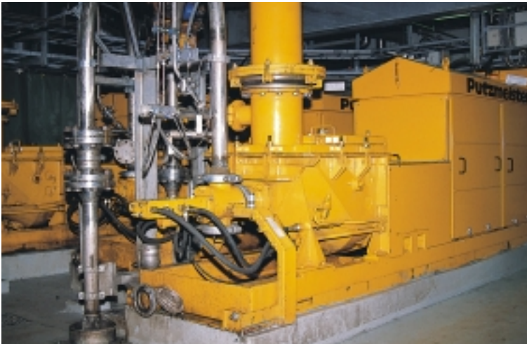
KOS 1070 coal sludge injection pump
