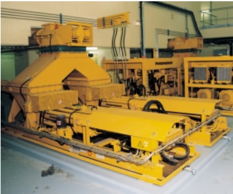
Sewage sludge reception silo with four KOS 1040's at Sarcelles, France
