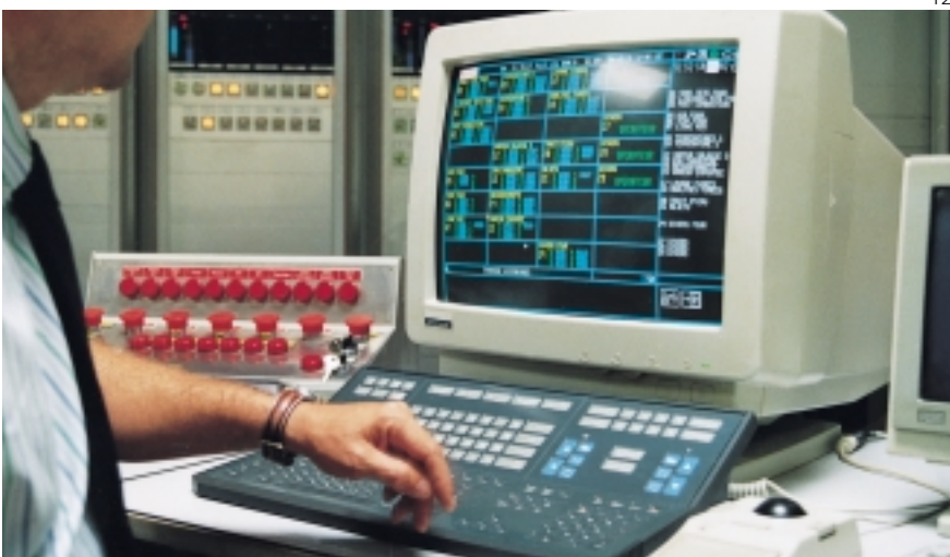
Central control console of a hazardous waste treatment plant which controls the entire incineration process
